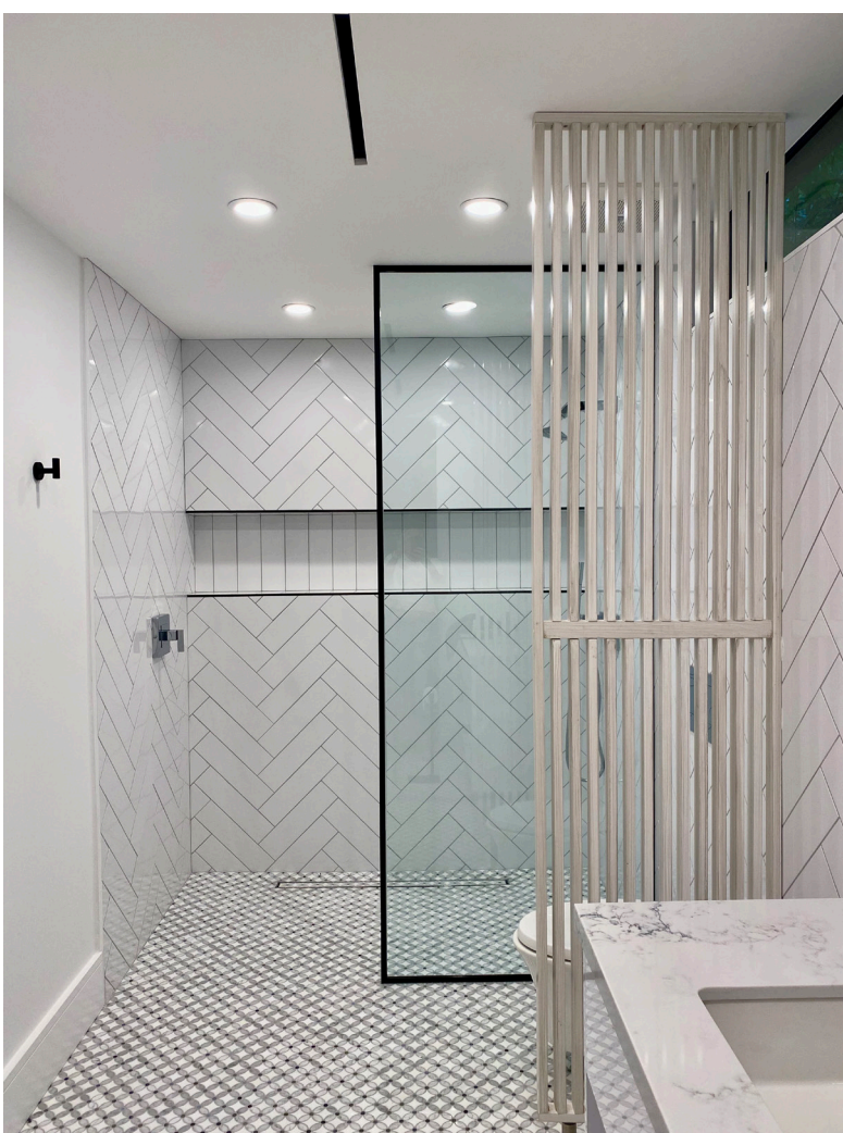
This previously beige and gold bathroom was transformed into a modern black and white space with a California vibe.
